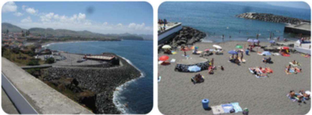
*Figure 4. Public beach at Ribeira Grande. (a) Emerged breakwater to protect swimming pool. (b) Pocket beach formed by sediment trapping. From Ng., et al 2014*
