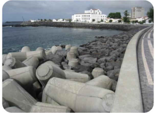
*Figure 6. Tetrapods line the boardwalk buffer zone to absorb wave energy. From Ng., et al 2014*
