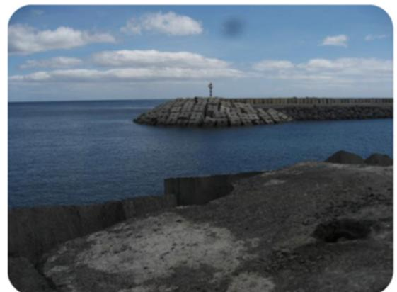
*Figure 5. Antifer cubes line the breakwater at the outer port to absorb wave energy. From Ng., et al 2014*
